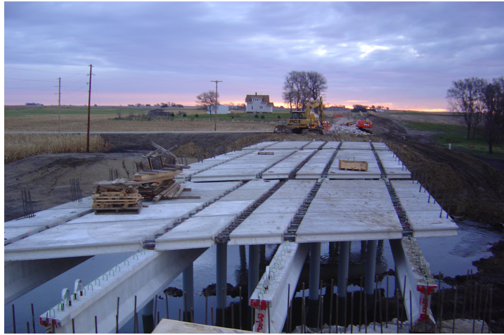
Figure 32. View of precast deck panel installation at Boone County Bridge
