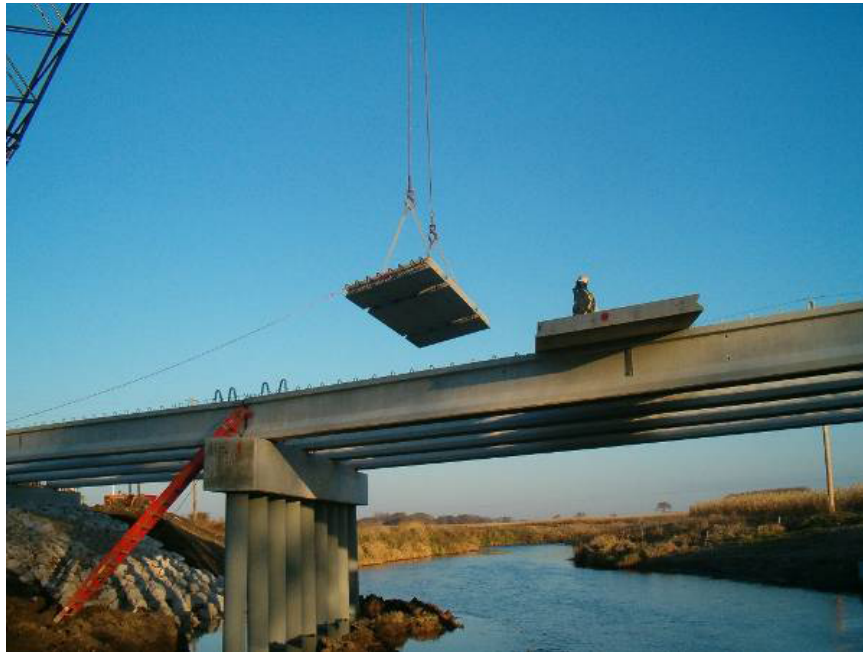
Figure 6. Installation of a precast concrete deck panel
