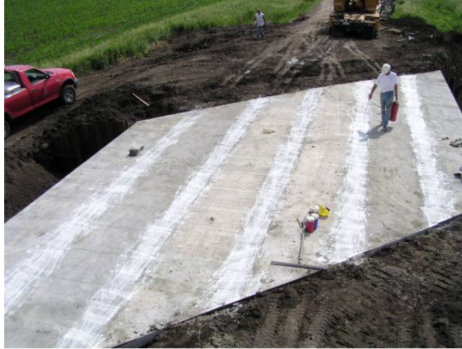
Figure 13. Black Hawk County Bridge near completion
