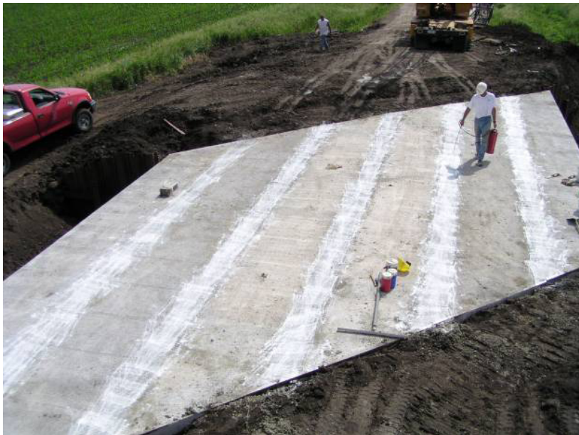
Figure 27. Black Hawk County Bridge near completion
