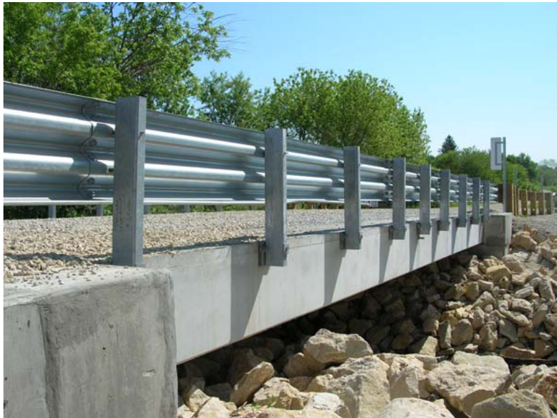
Figure 35. Completed Madison County Bridge
