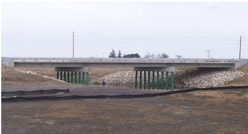
Figure 1.45 Completed replacement bridge on 120th St
