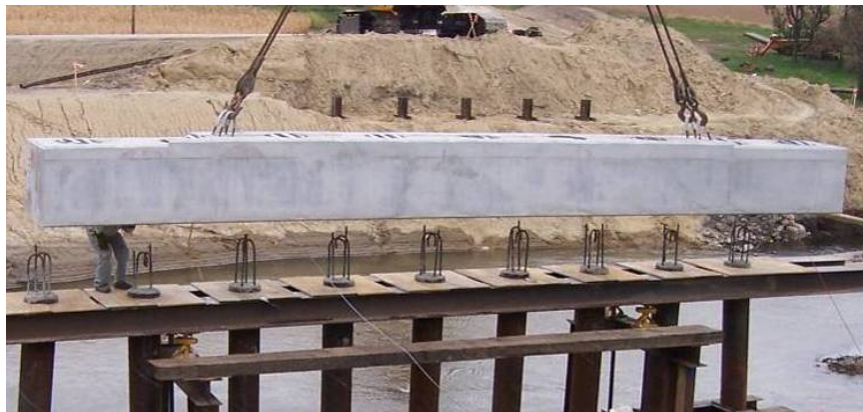
Figure 30. Installation of precast pier cap at Boone County Bridge
