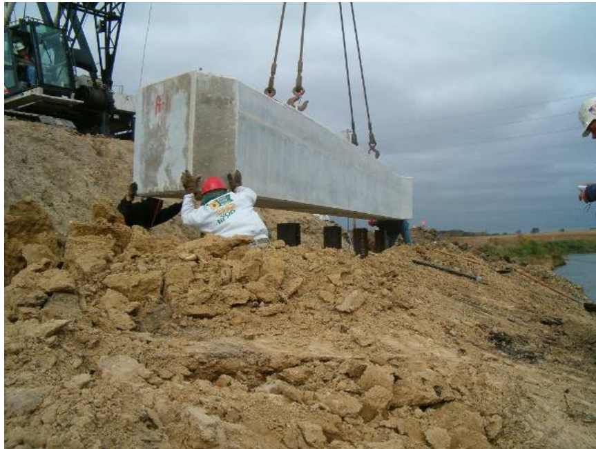
Figure 5. Placement of precast abutment cap onto H-piles
