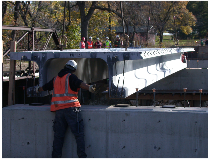
Figure 19. Installation of precast concrete pi-girder
