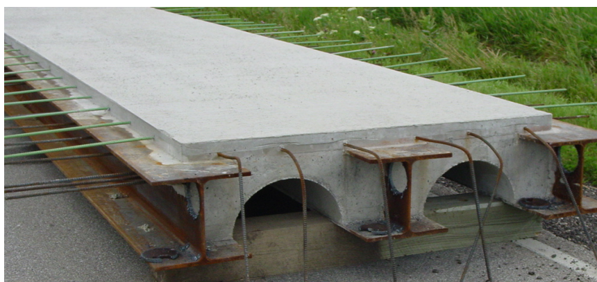
Figure 24. PMBISB system deck panel used on Black Hawk County Bridge
