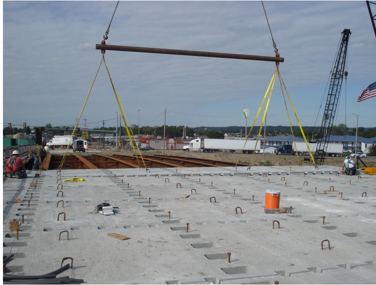
Figure 43. Installation of precast deck panel at 24th Street Bridge
