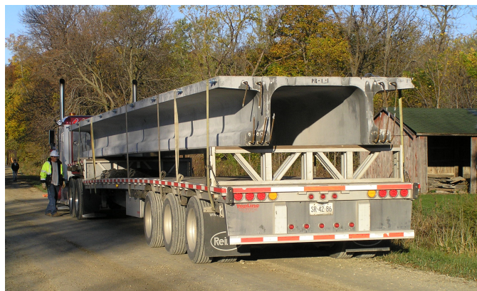
Figure 18. Delivery of a precast concrete pi-girder
