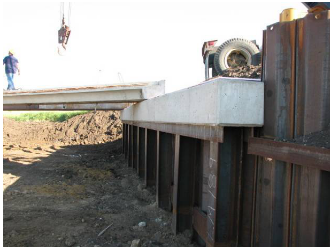
Figure 12. Precast concrete abutment cap supported by steel H-piles
