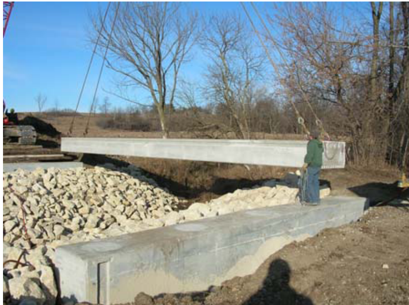
Figure 39. Installation of precast box beam at Madison County Bridge
