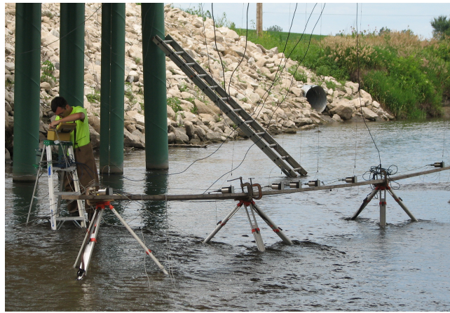
Figure 2.3 Tripod system used to support displacement transducers
