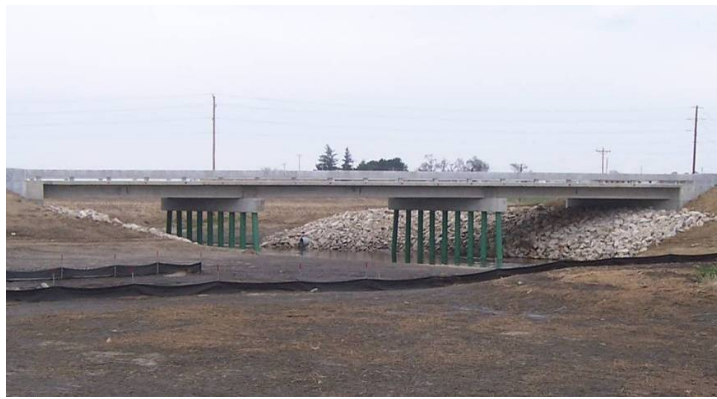
Figure 28. Completed Boone County Bridge
