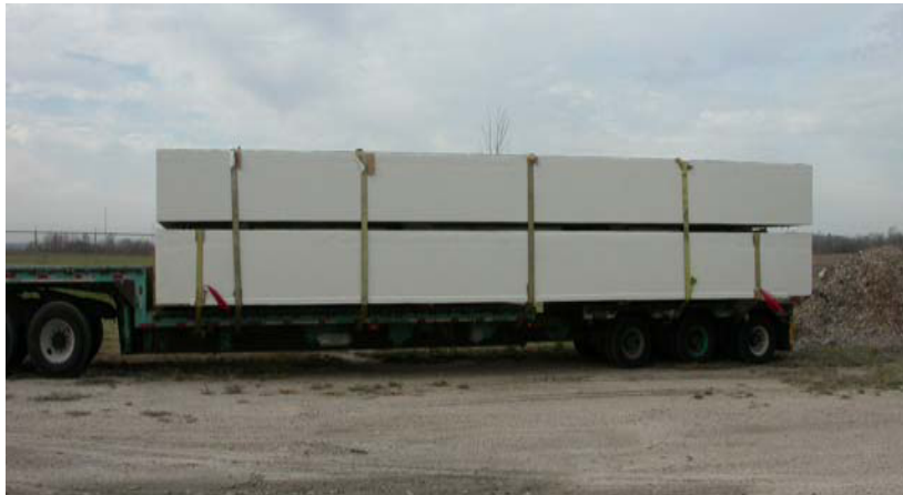
Figure 9. FRP panels loaded onto truck trailer for delivery
