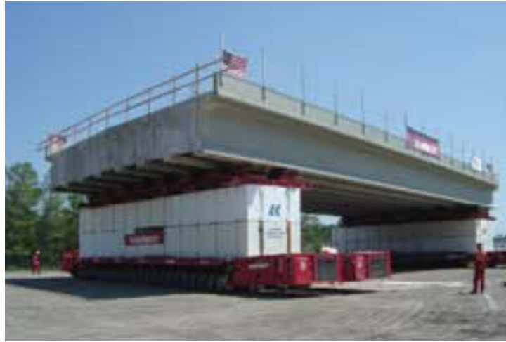
Figure 20. SPMTs used to transport an entire bridge superstructure
