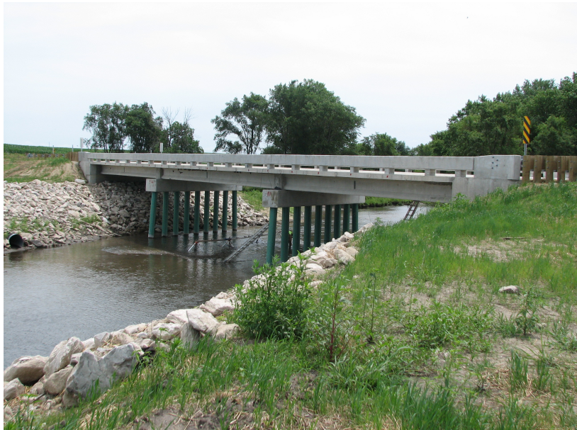
Figure 1. View of completed Boone County Bridge
