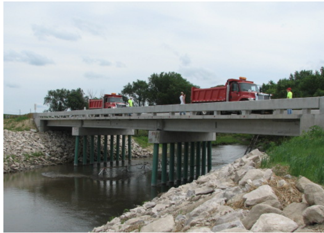
Figure 2.12 Static test (Load Case 2)
